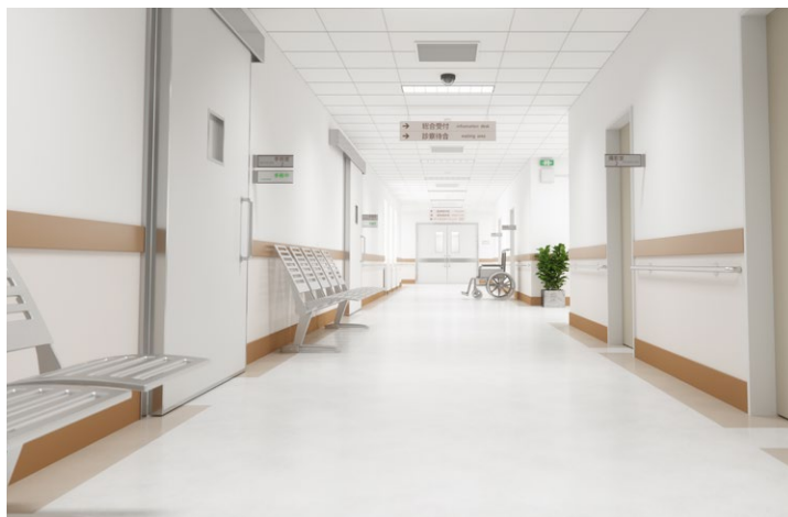
In corridors with a lot of traffic, the walls and corners quickly get worn down.
