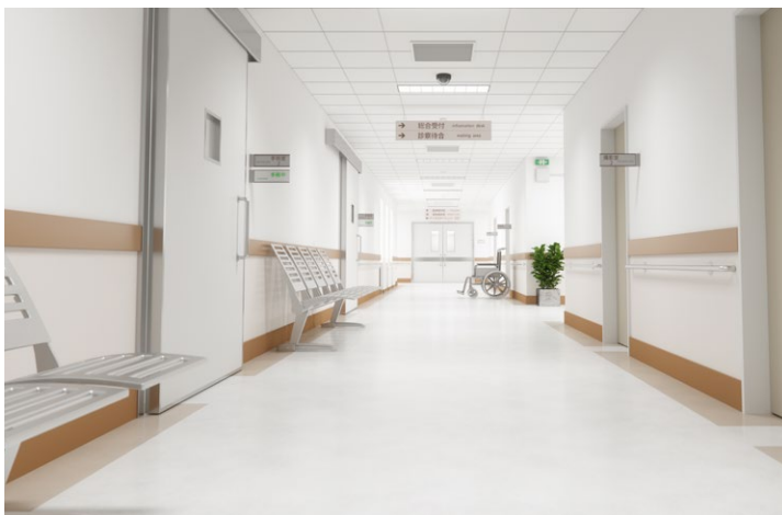
In corridors with a lot of traffic, the walls and corners quickly get worn down.
